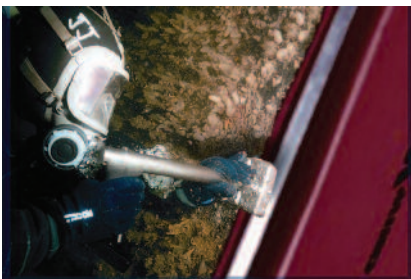
Diver attaching a patch to a hull
